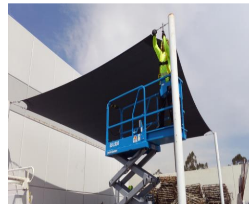
After Photo of the Replacement Project
