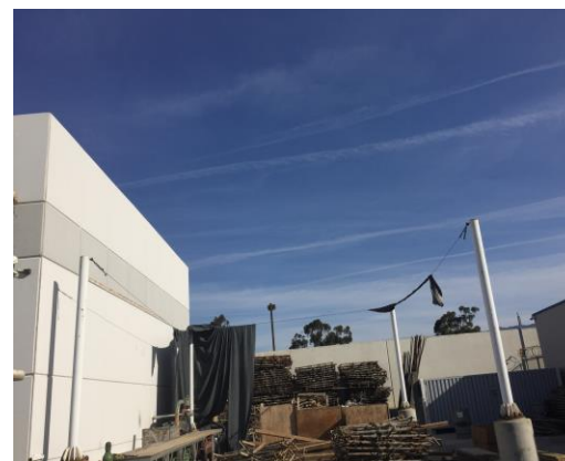
Before Photo of the Replacement Project
